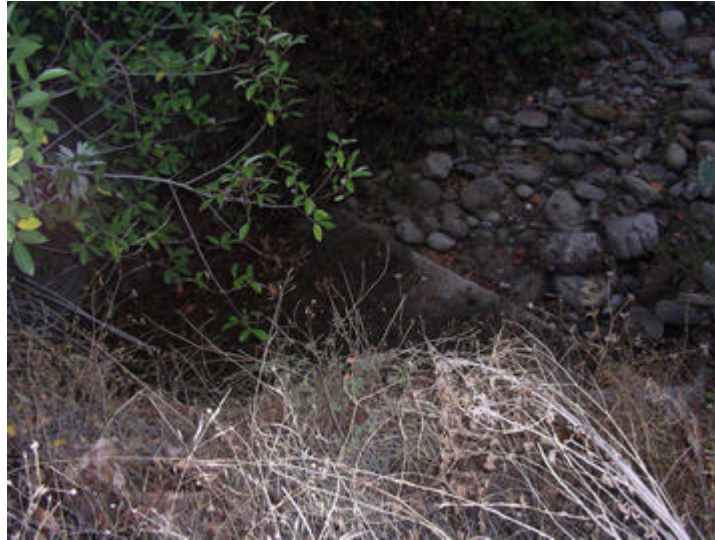
Concrete apron at upstream end of culvert
