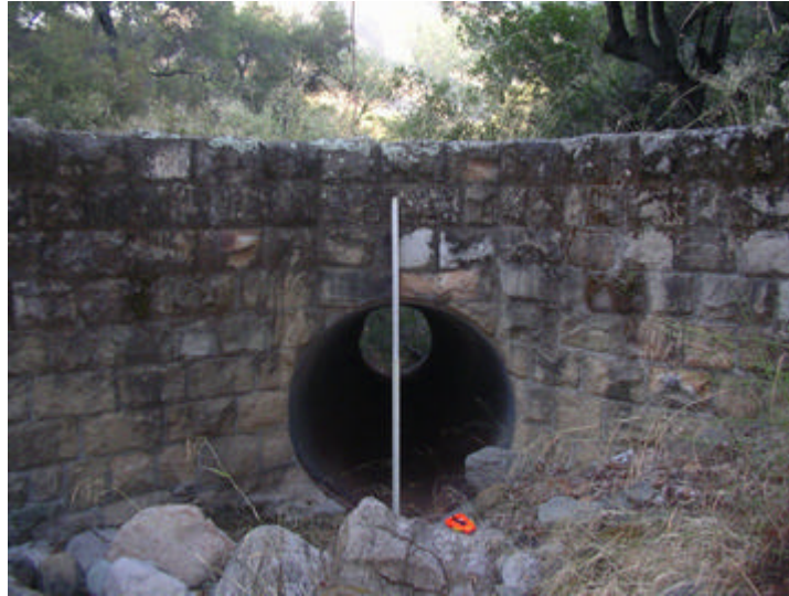
Looking downstream at corrugated metal culvert
