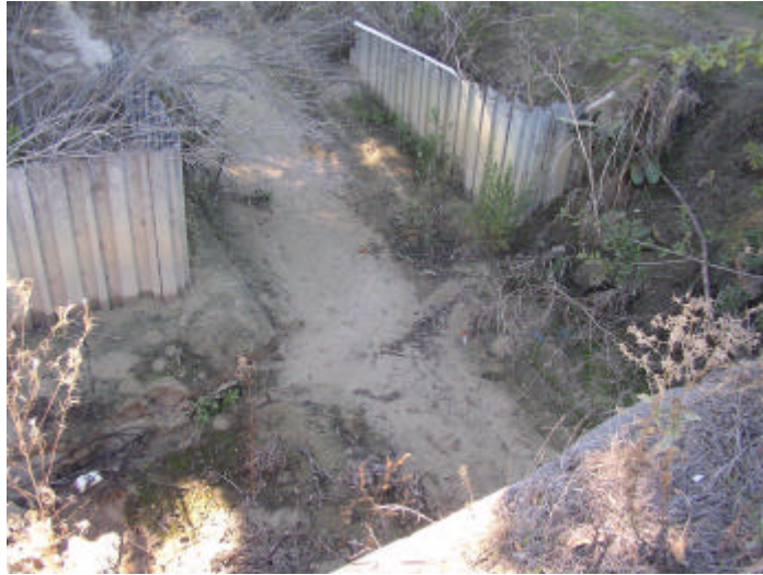
Metal revetment downstream from culvert
