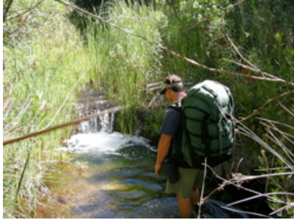
Scour pool 950 feet upstream of dam
