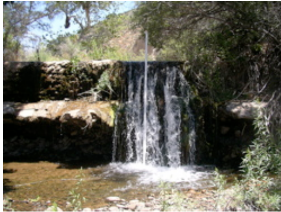
Horse Creek Dam
