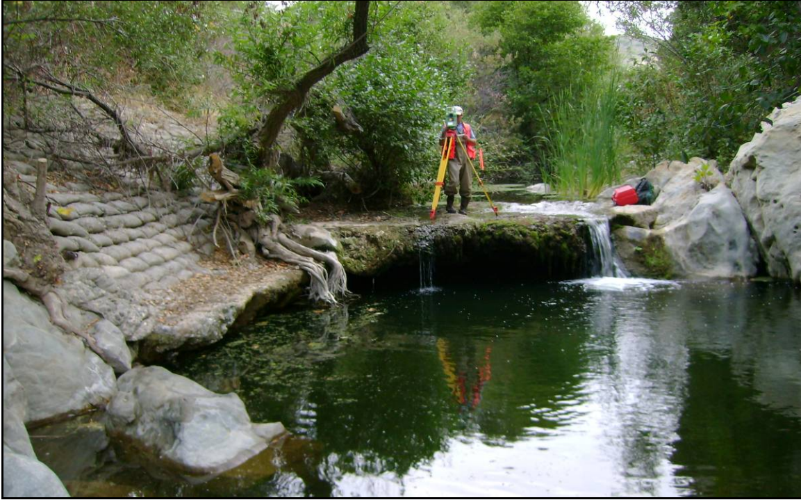
Figure 4.22 - GA13 is keyed into the sacrete wall and large boulders and exposed bedrock. There is ample evidence of scour along the undercut wall and GA13 is undercut approximately 5 ft. The pool elevation is controlled by a bedrock chute the spans the entire width of the downstream channel.
