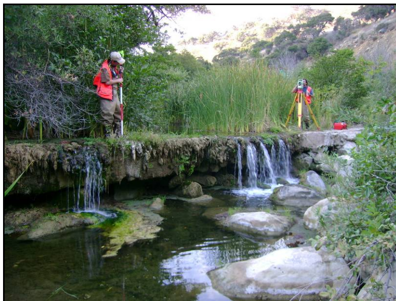
Figure 4.15 – GA 7 is skewed at a 45-degree angle with the centerline of the channel. It is likely that this structure was built to protect a now- abandoned pipe that is visible in parts of the structure.
