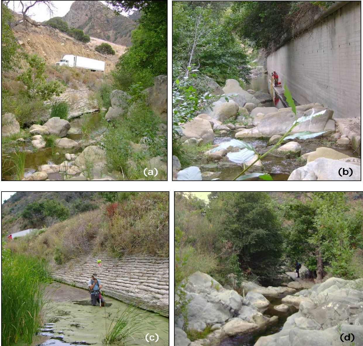
Figure 5.7 - Upper reach, from downstream to upstream, consists of (a) boulder steps and boulder cascades followed by long glides, highly confined banks due to the proximity of the highway (b and c), followed by a section of channel bed controlled by bedrock (d) and concrete grade control structures.
