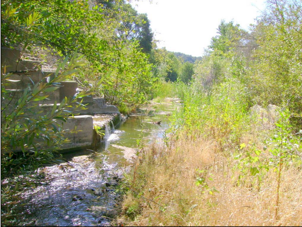
Figure 3 – Outlet of Las Canovas Creek culvert, at the confluence with Gaviota Creek. Looking downstream towards tailwater control in Gaviota Creek.
