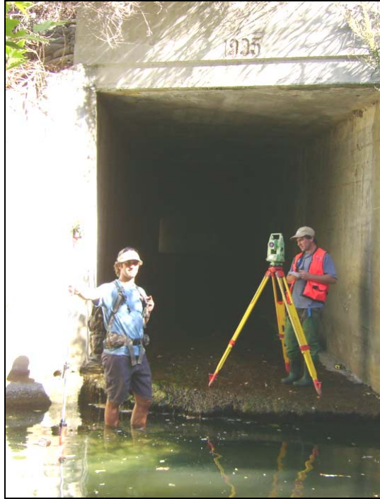
Figure 5 – Outlet of Upper Gaviota Creek culvert.
