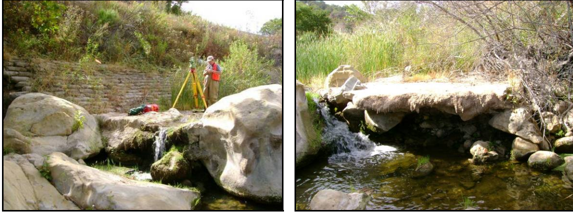
Figure 4.18 – GA8 appears to be a concrete apron less than 1 foot thick, poured over an existing boulder cluster. It is undercut approximately 4 ft and failing around the large mid channel boulder.
