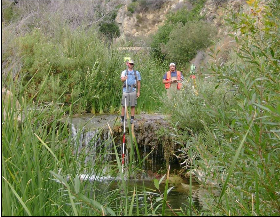
Figure 4.7 – Looking upstream at GA4, which is controlled by a boulder weir constructed by CA State parks. GA4 is undercut approximately 3 ft and the banks and pool are scoured and have been reinforced by large rock placed along the highway revetment.
