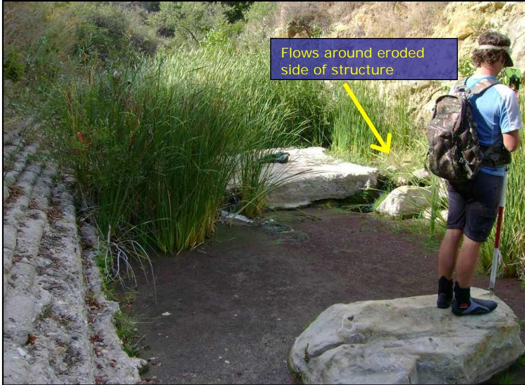
Figure 4.20 –GA10 is failing along the river-left bank from flanking that has eroded the native material along the steep right bank.
