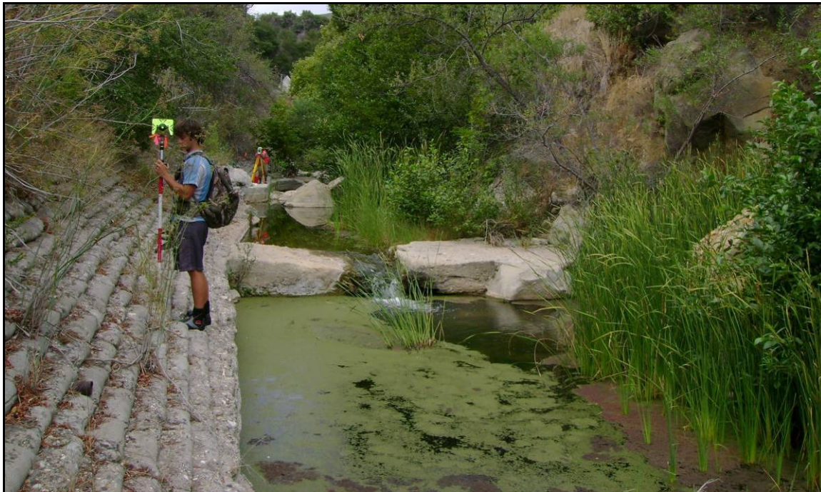
Figure 4.21 – GA11 and GA12 are keyed to sacrete and large boulders.
