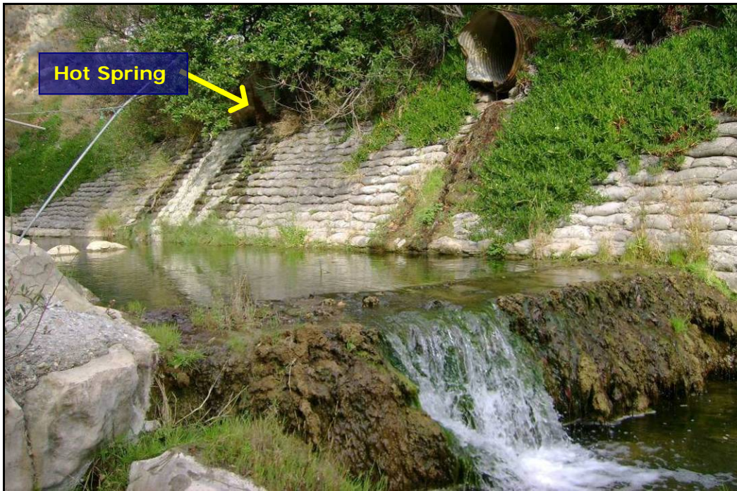
Figure 4.8 – Grade control GA5 located 80 ft upstream of GA4. Note the 36-inch highway drainage culvert and hot spring outlet located at the top of sacrete revetment wall.
