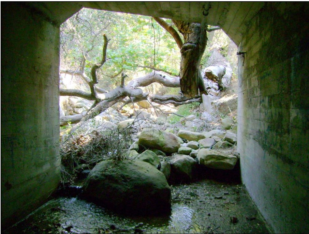
Figure 4 - Looking upstream through the inlet of the Highway 101 Las Canovas Creek culvert. The crossing is a 10 ft x 10 ft box culvert, with 3 turns and four distinct breaks in slope. There is substantial aggradation of boulders and cobbles at the inlet.
