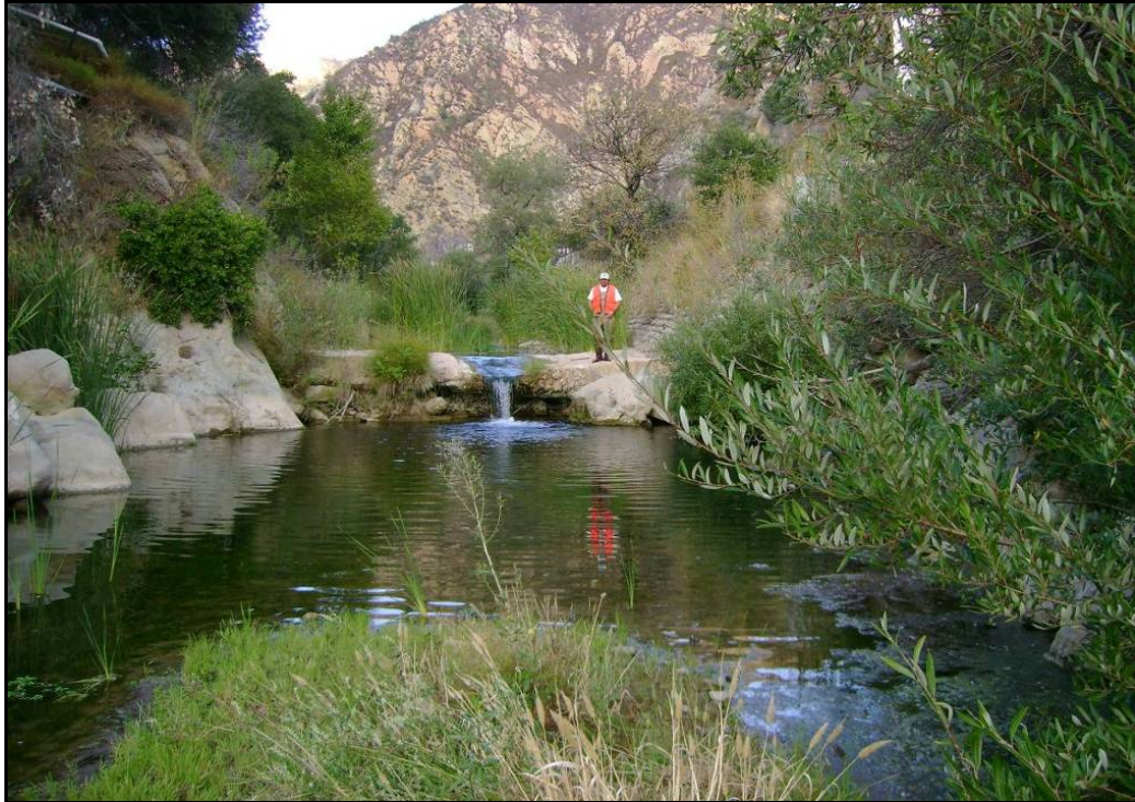
Figure 4.2 – Looking upstream at grade control GA2. The structure is anchored to the concrete revetment wall (right side of photo) and to exposed bedrock on the other side. The tailwater pool was one of four large pools found in the study reach.
